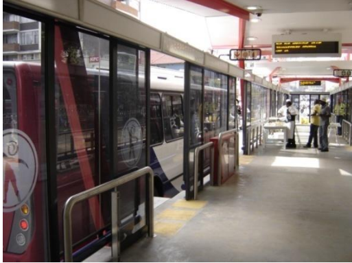
A typical BRT station
